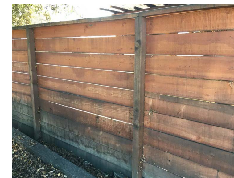
WOOD SCREEN FENCE AND GATE
